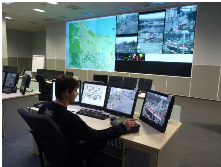
Operation room in the Traffic Management Center in Gdańsk
