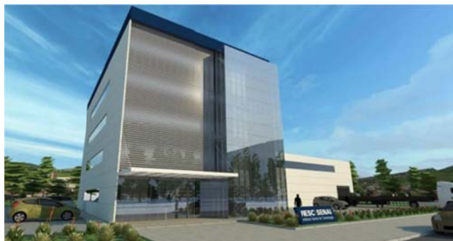
Picture 4 – Digital plant of Instituto SENAI de Tecnologia
